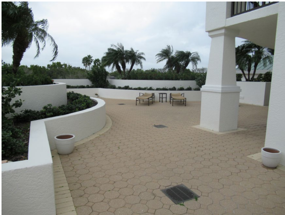
View of exterior terrace unit 403.
