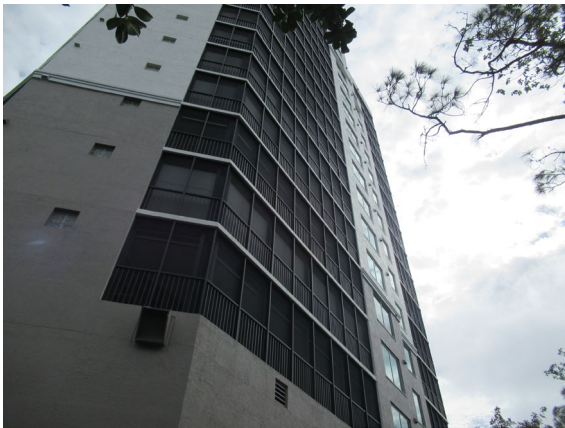
Partial view of southern façade.
