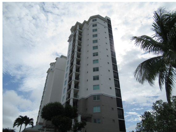
View of western facade.
