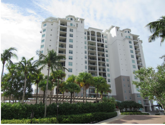
View of northern facade.
