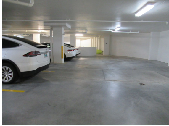
General view of the covered parking area.
