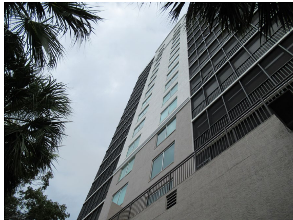
Partial view of southern façade.
