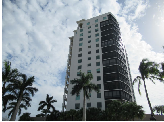
View of western facade.
