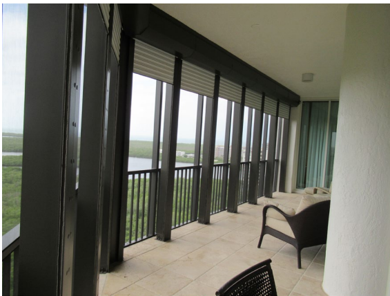
View of balcony with ceramic tile and shutters unit 1802.
