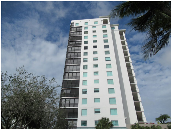
View of the eastern facade.
