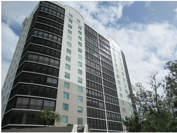
Partial view of southern facade.
