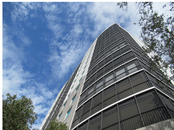
Partial view of southern facade.
