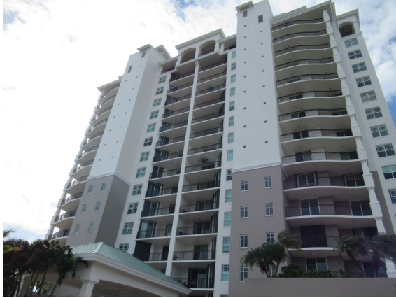
View of northern facade.
