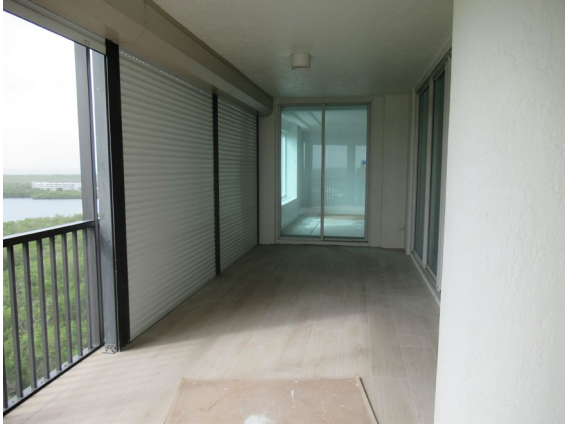
View of balcony with ceramic tile and shutters unit 1404.
