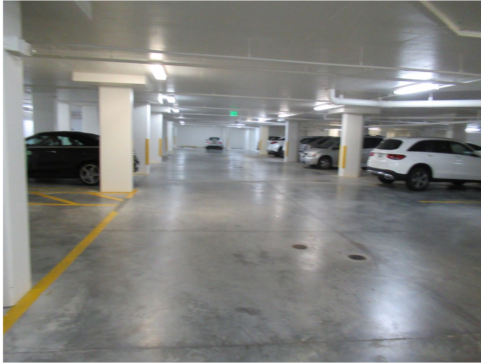
Photo 11 – Partial view of the covered parking area.
