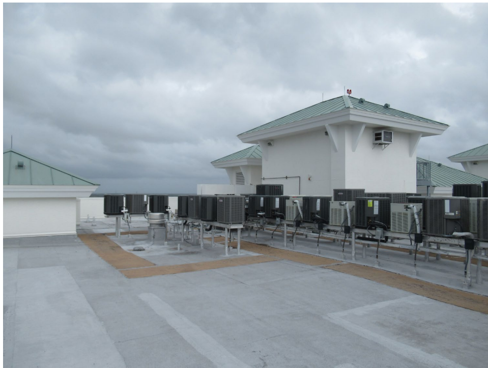
Photo 6 – View of roof section and HVAC equipment.
