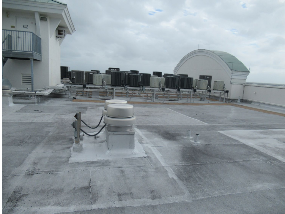
Photo 5 – View of roof section and HVAC equipment.
