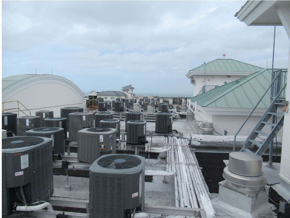
Photo 5 – View of roof section and HVAC equipment.
