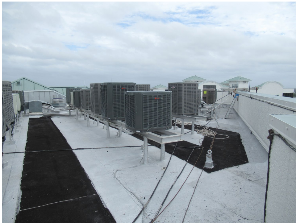
Photo 6 – View of roof section and HVAC equipment.
